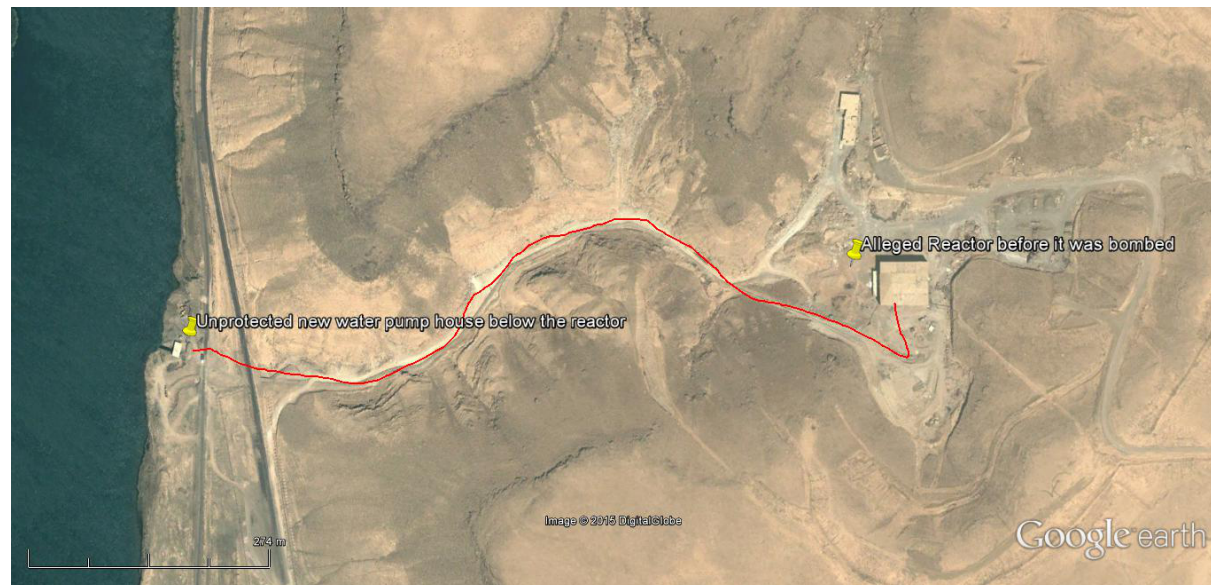
Figure 4. The new unprotected pump house would pump water up hill to the building according to IAEA. The pipeline passes under two right-of-ways without fencing or protection. The better road to the site leads from the DWTP and not up the canyon from the river. There is no major security checkpoint on either road leading to the building, a building which supposedly housed a reactor core load of uranium fuel.
