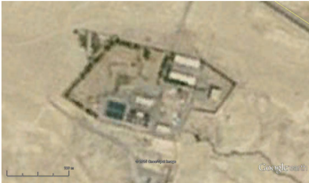
Figure 1. The Desert Water Treatment Plant is well established even in 2004.
