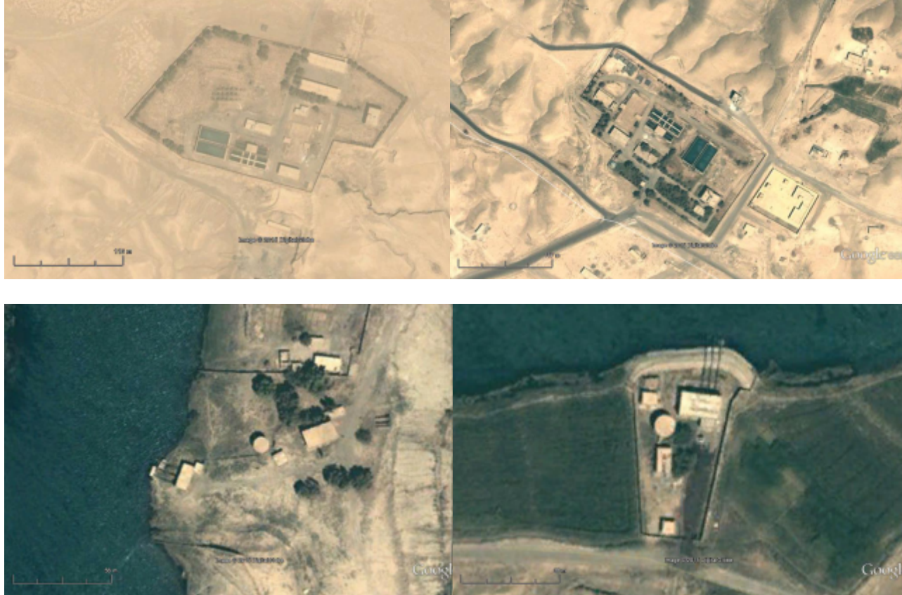
Figure 5 The DWTP and its riverside pumping station are visible on the left and the nearly identical Tibni water treatment plant is on the right. Clearly they were built from the same engineering drawings
